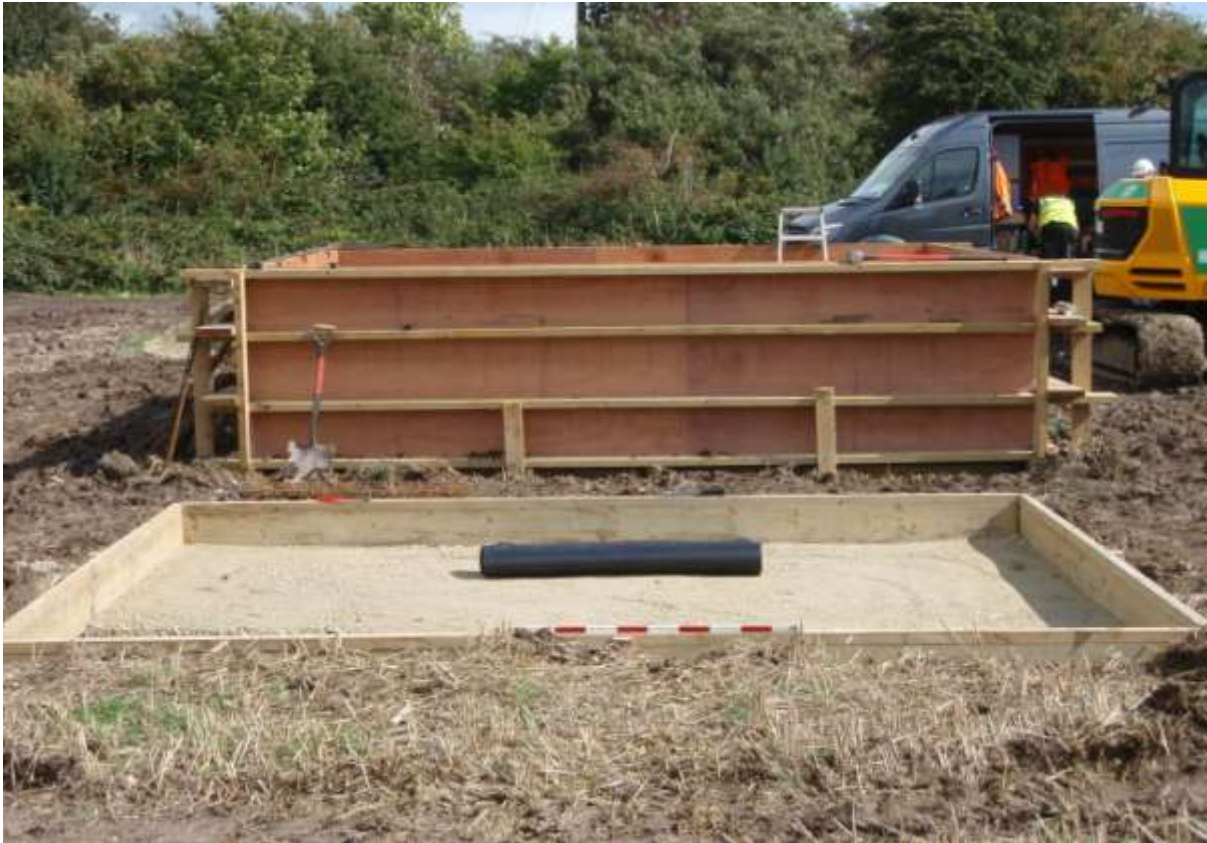
Plate 7. Construction of the Inverter base which sits within the topsoil
