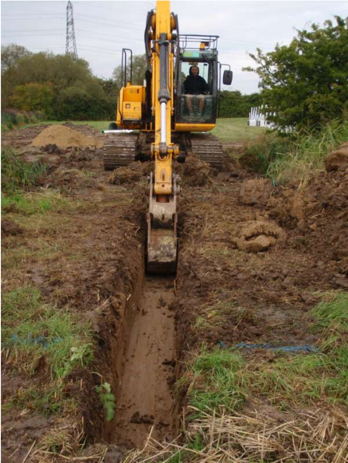
Plate 6. Cutting the AC cable trench (toothless bucket)
