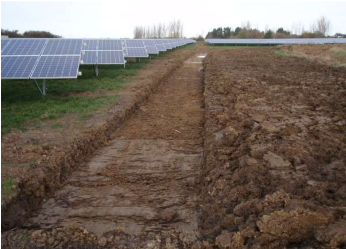
Plate 8. Construction of the Swales (drainage ditches)
