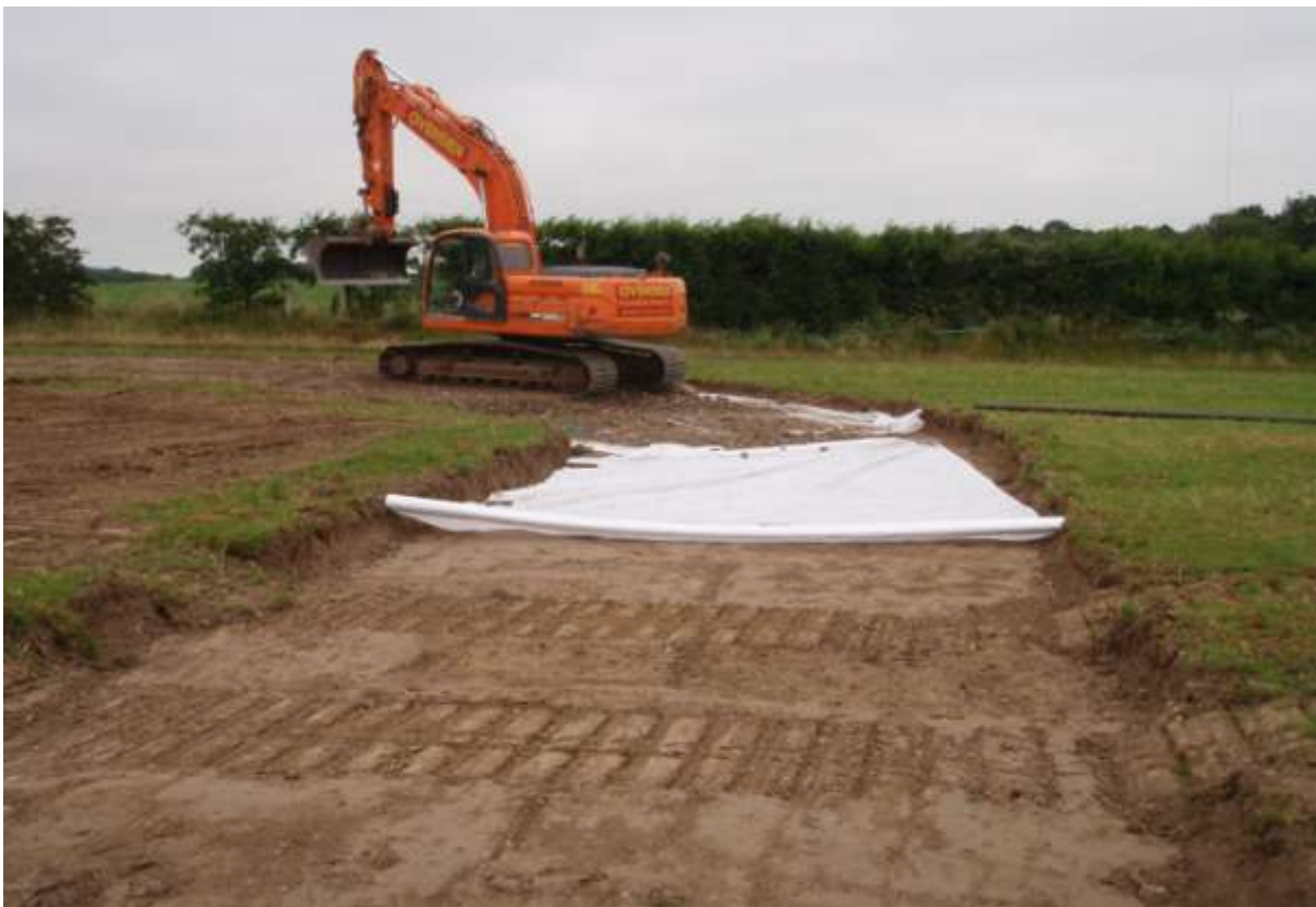
Plate 3. View showing soil reduction for maintenance road
