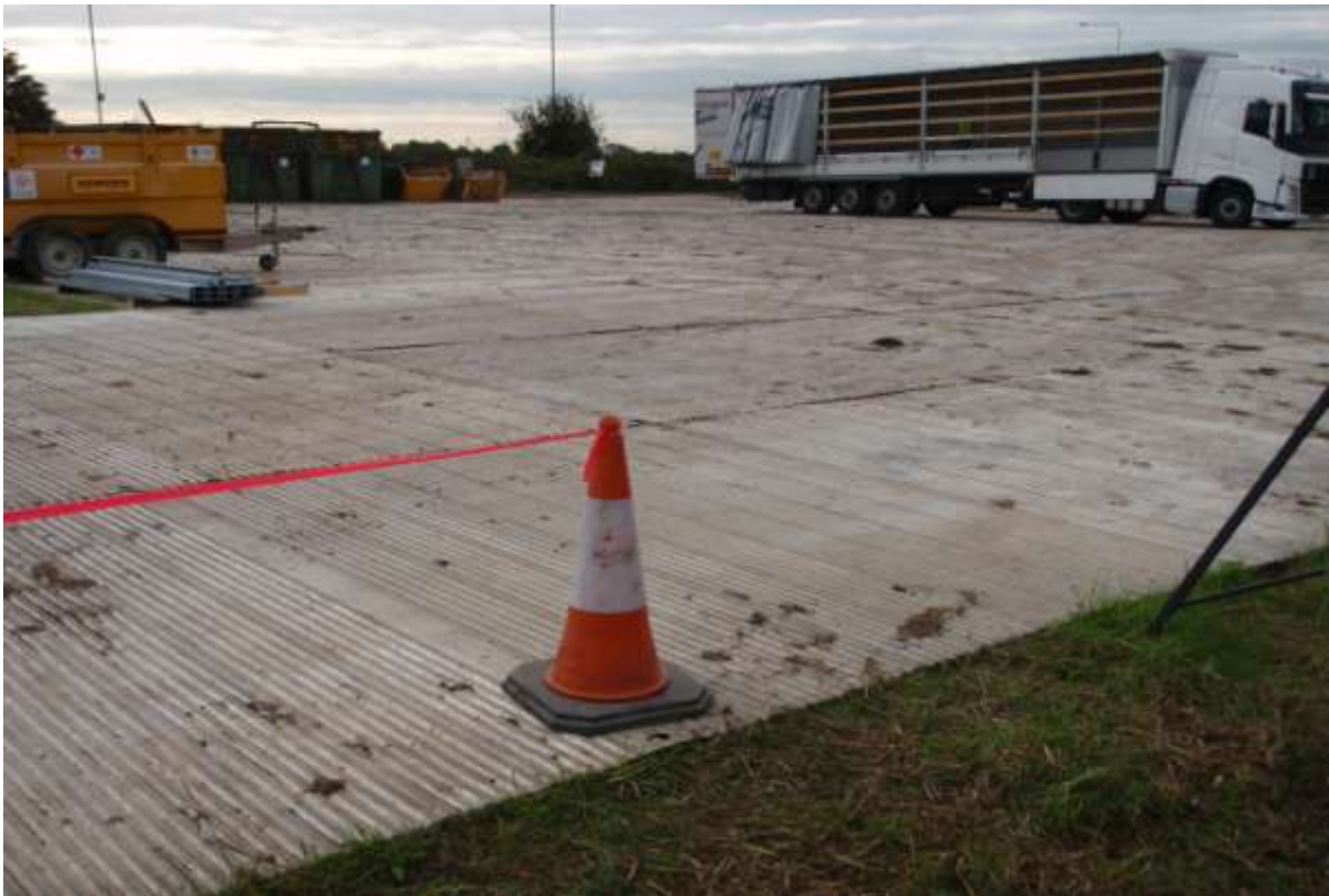
Plate 2. General view of site compound showing galvanised sheeting
