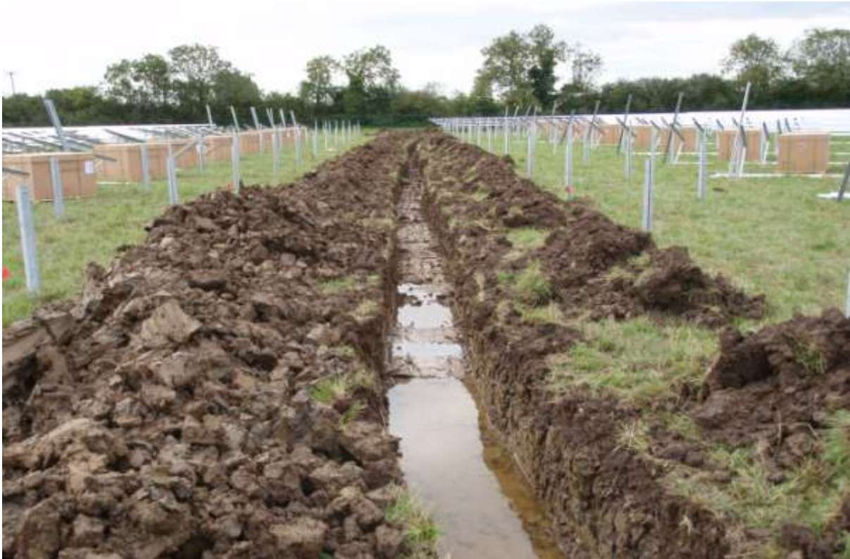
Plate 4. The site showing cutting of main cable trench
