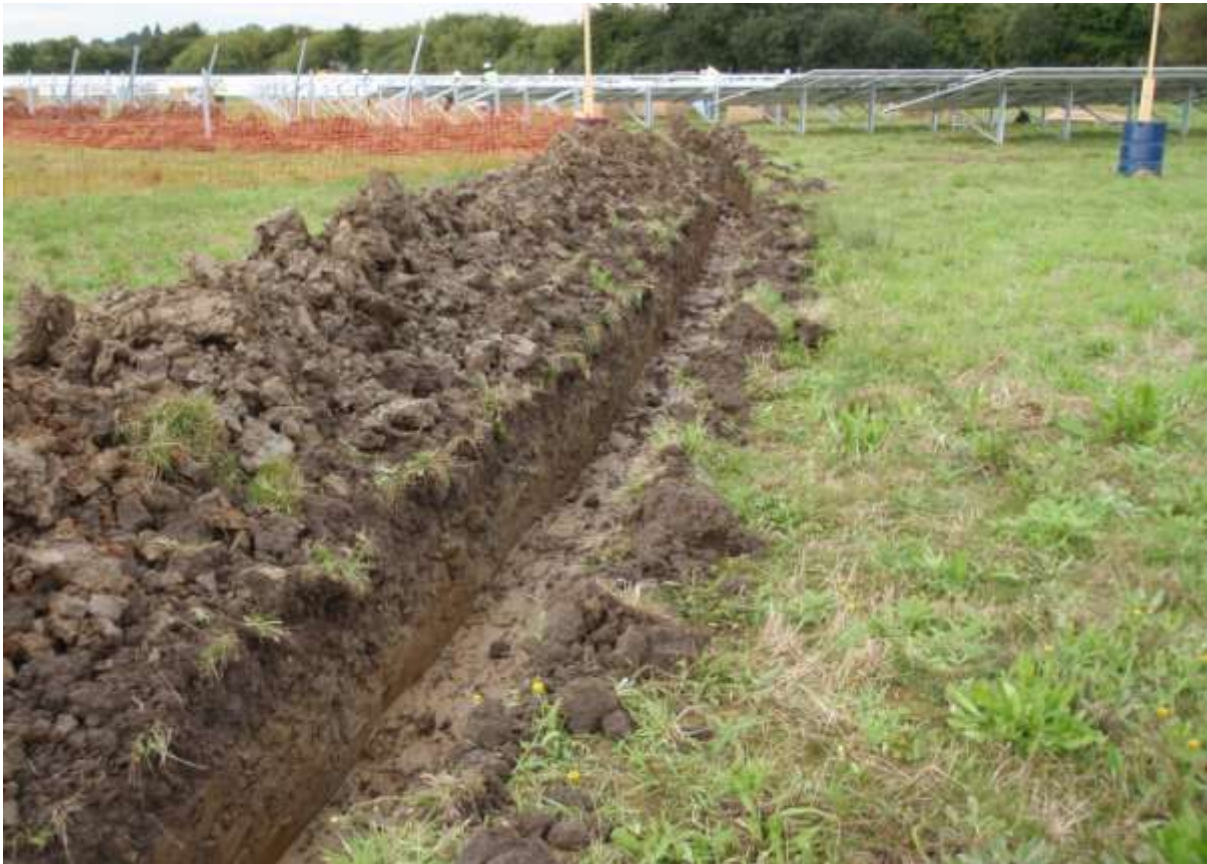
Plate 5. The AC cable trench
